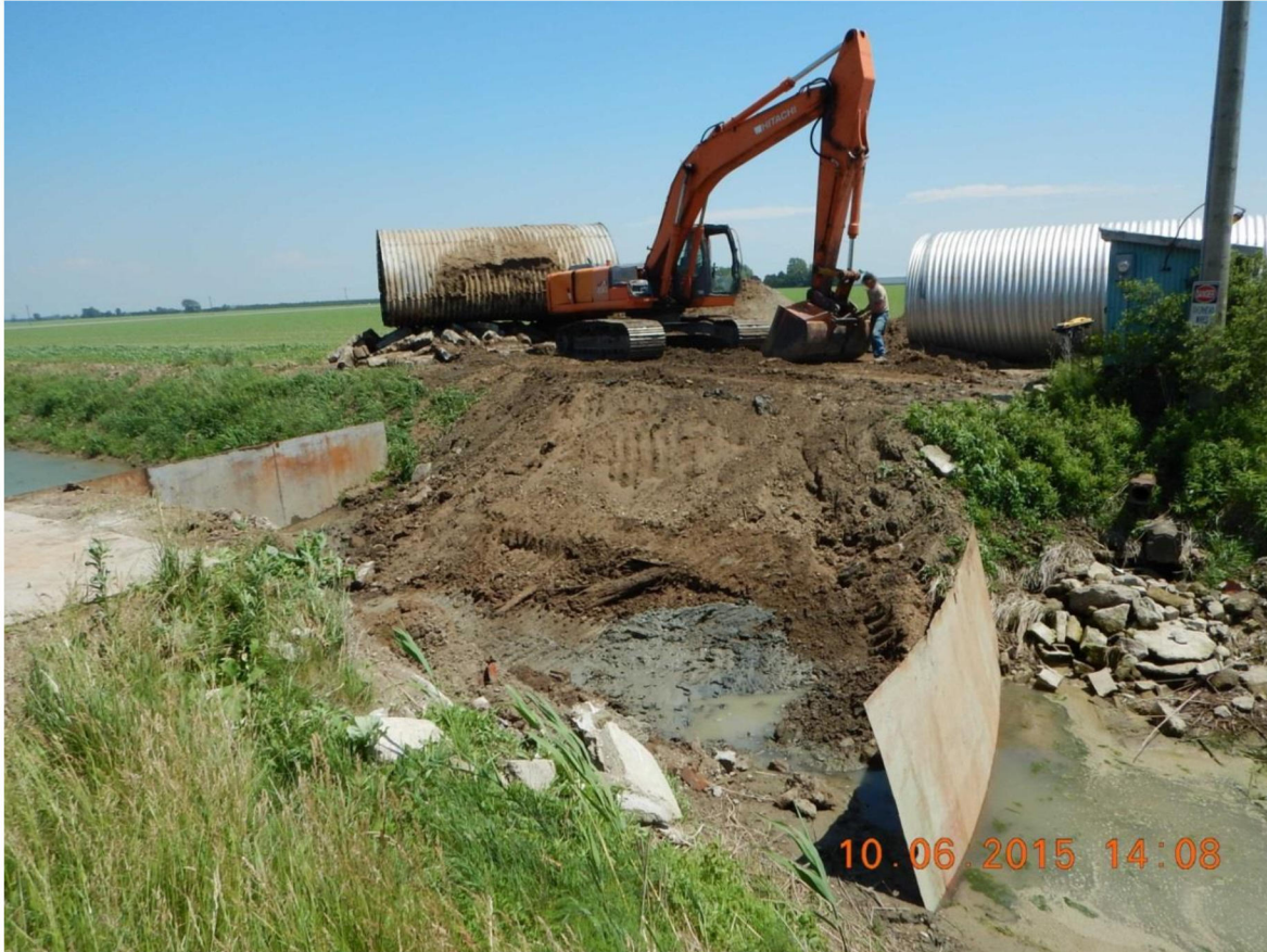
Figure 2. Isolation of Site
