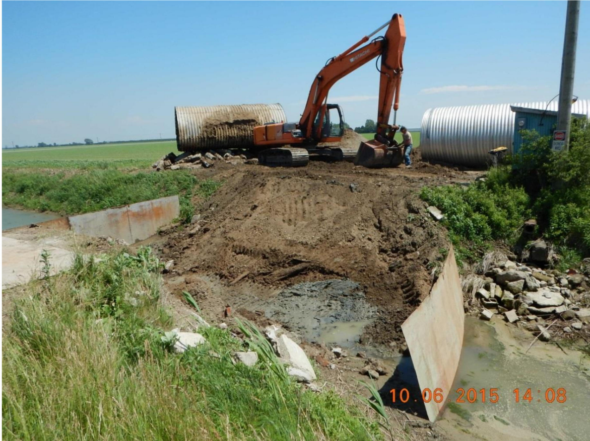
Figure 2. Isolation of Site
