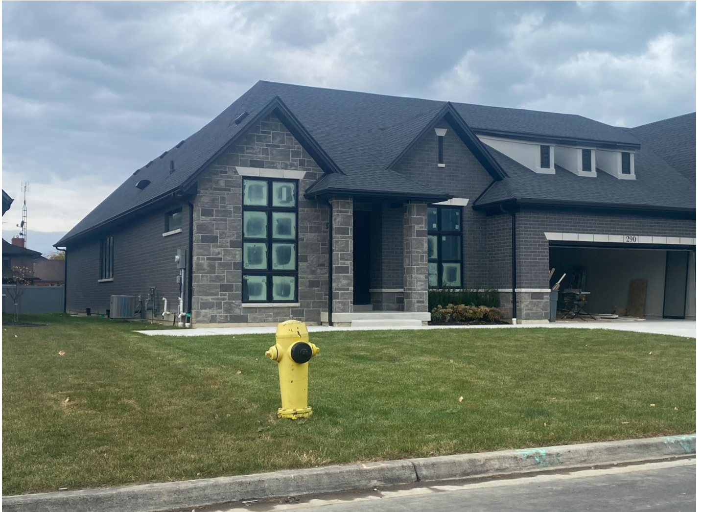
Air Conditioning Encroachment Example – 290 Xavier Circle Photo taken on November 4, 2024
