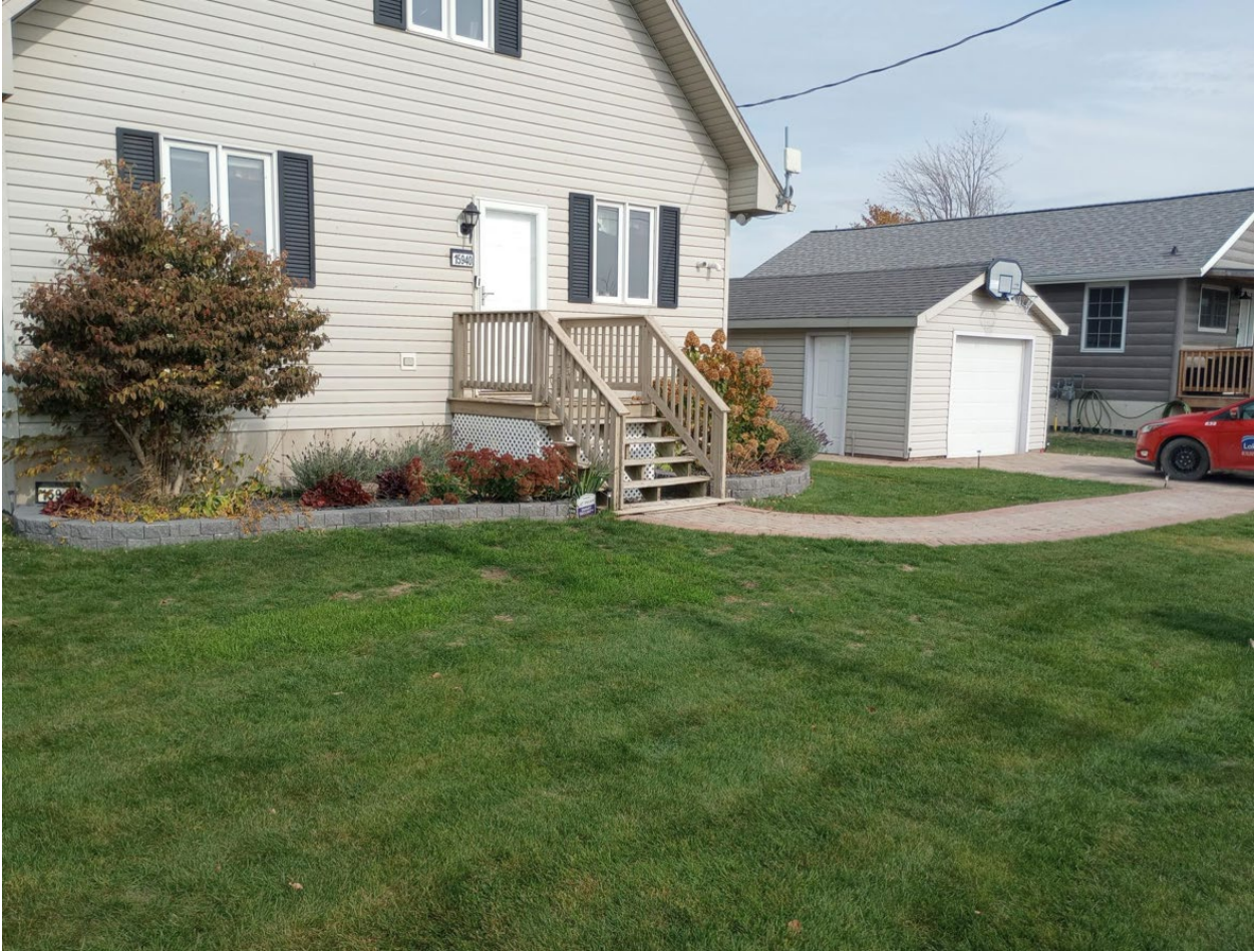
Picture looking northeast at the subject property from the road
