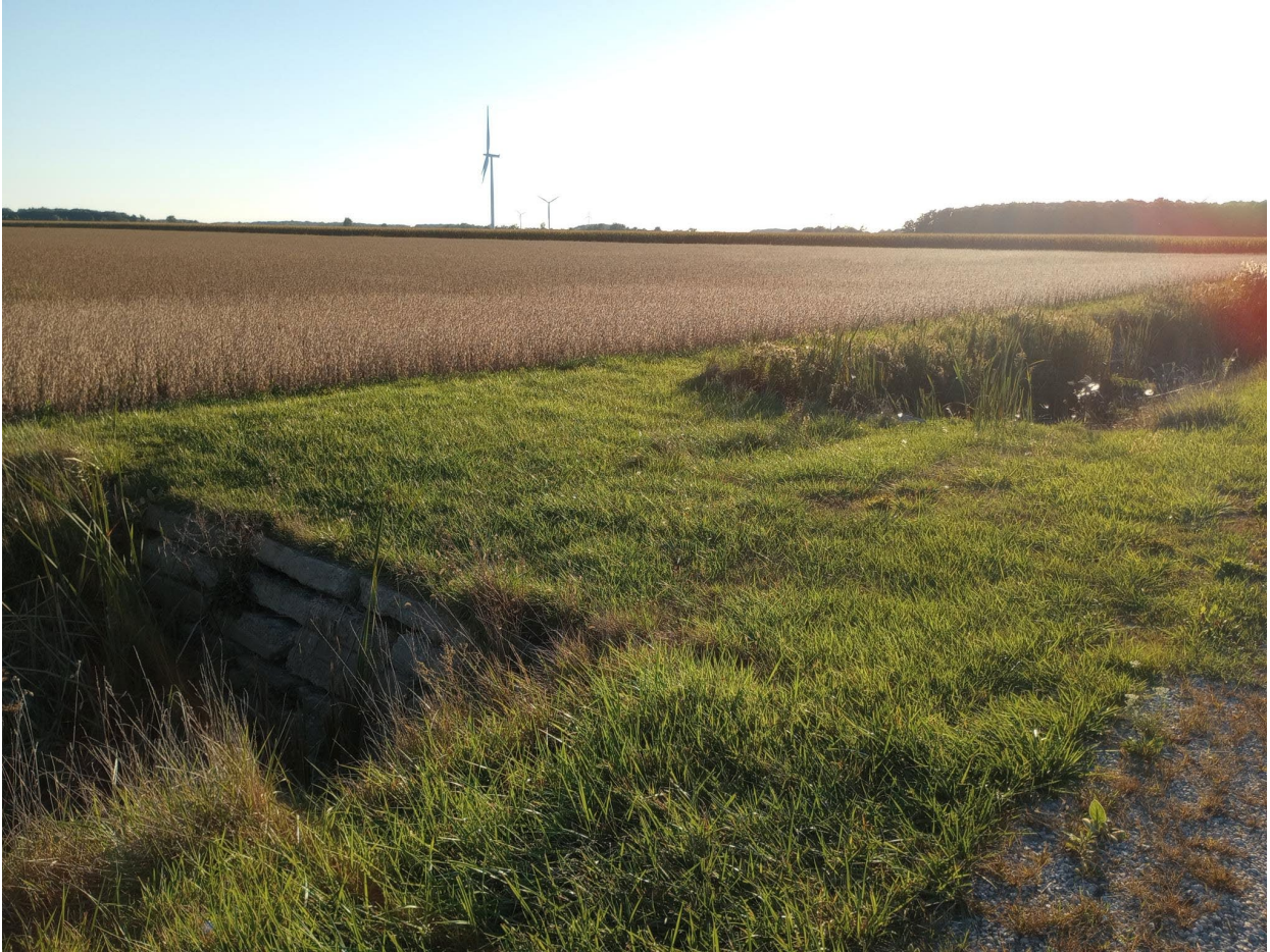
Picture of access bridge to the farm property located on the west half of the farm taken from the street
