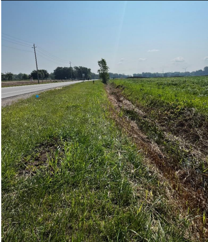
Looking downstream in an easterly direction at the Bernard Tellier Drain along the south side of County Road 2.
