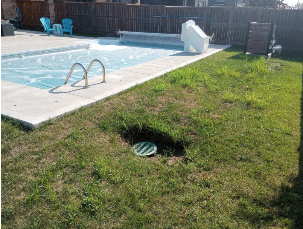
Figure 3: Existing drain in rear yard, located between pool and rear lot line.
