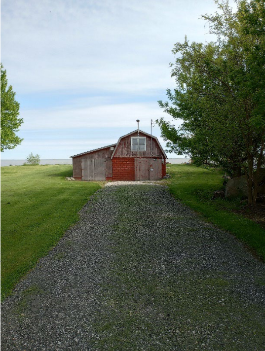
Figure 1: North-facing view of existing building from street.
