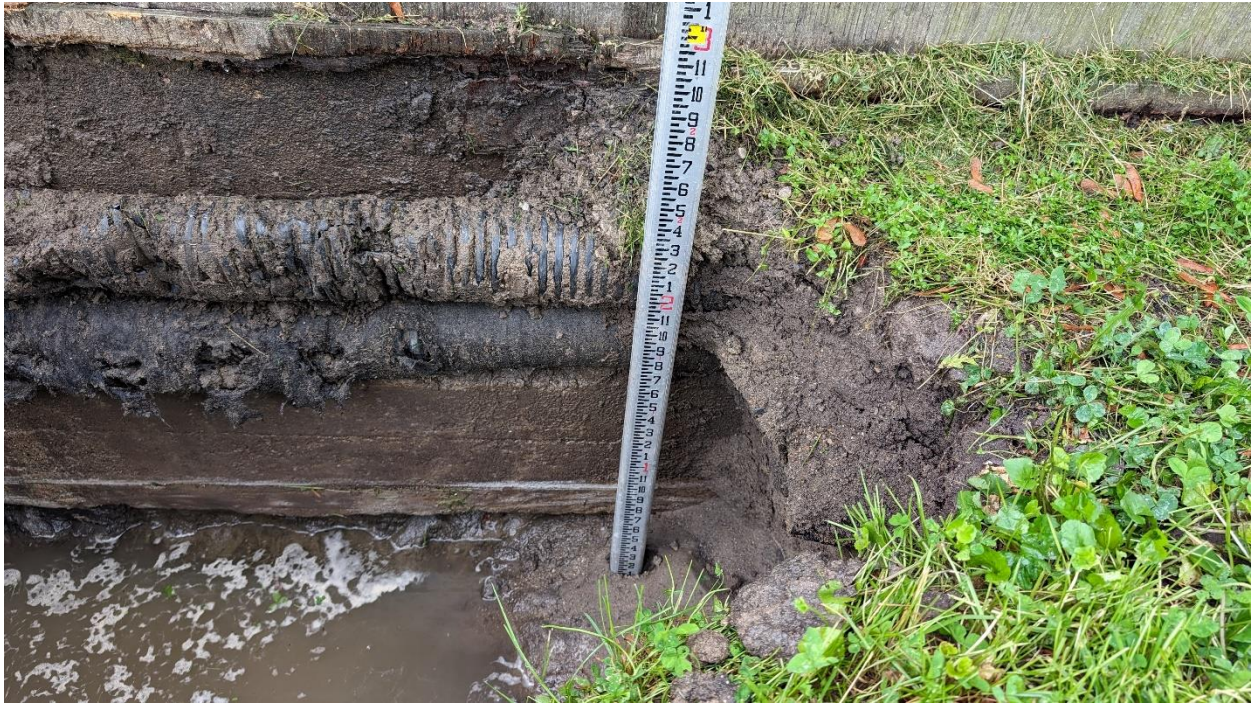
Figure 4 – Footing depth below grade.
