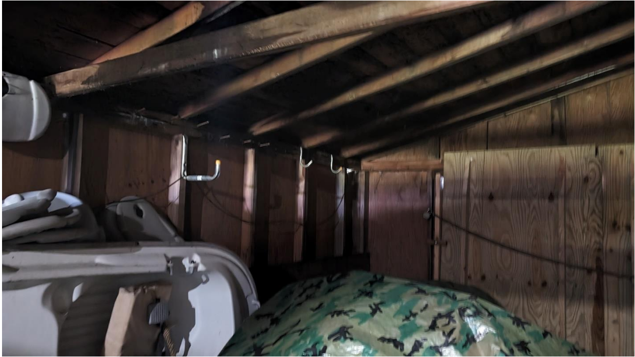
Figure 9 – Inside of the lean-to portion of the building.
