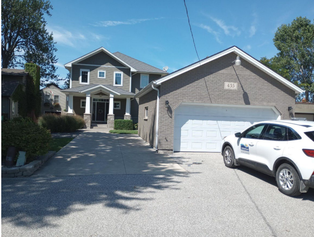
Figure 1: Existing accessory building and dwelling as seen from street, facing north.
