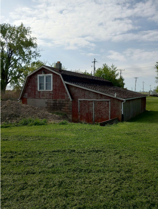
Figure 3: Rear view of existing building facing southeast.
