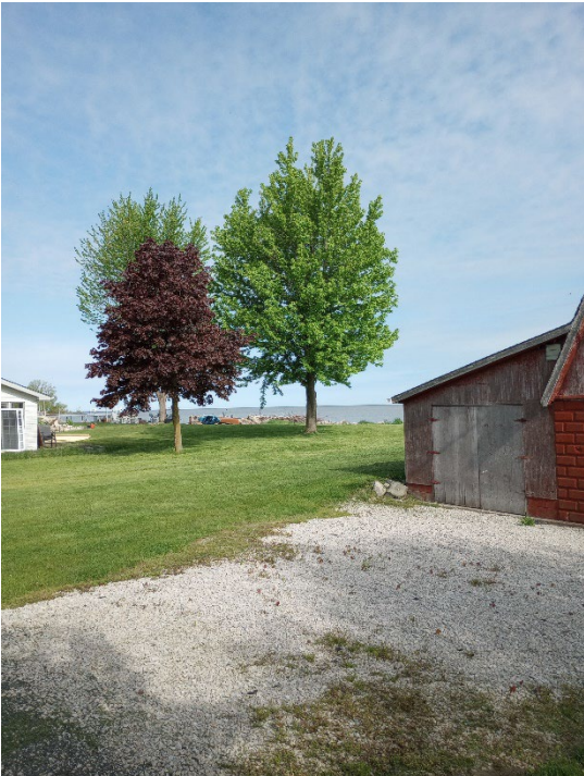
Figure 2: Northwest-facing view of existing building and property.
