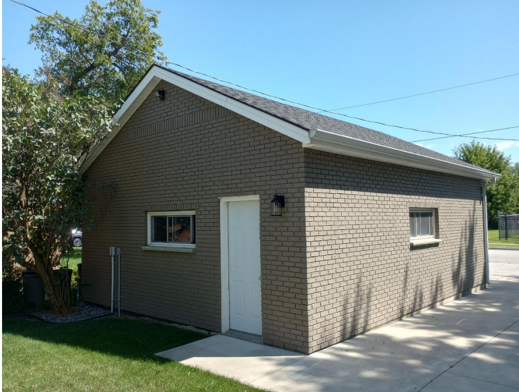
Figure 5: Rear and west sides of existing accessory building as seen from front yard of dwelling, facing southeast toward street.
