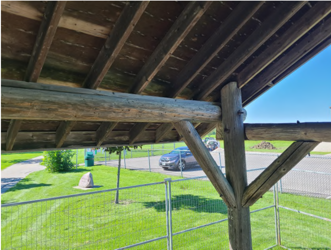
Photo #4: Typical Top-of-Post Connection
